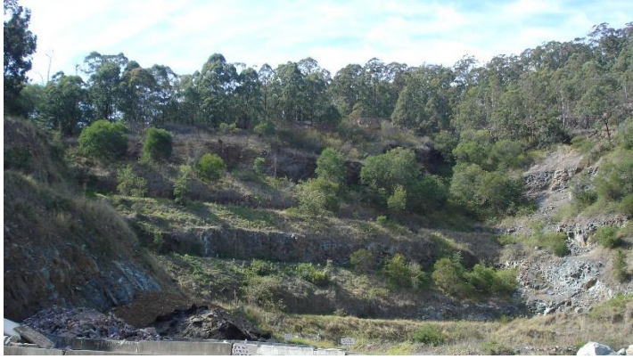
Rehabilitated completed benches above the Extraction Area A
